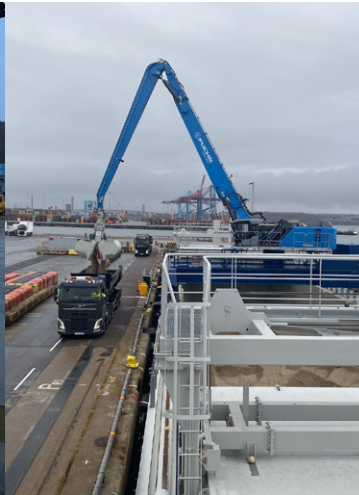
DISCHARGING SAND TO LORRIES
